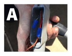
**A:** Connect the 'Pulse +' wire from your flow meter to the red wire (IN 1) on the Altrac cable. Connect the 'Pulse -' wire from your flow meter to the black wire (Ground) on the Altrac cable. Connect the foil shield to earth ground.
