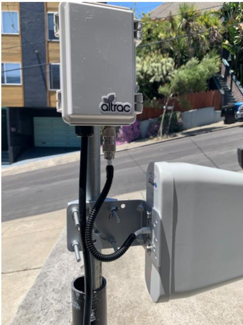
**NOTE:** The directional antenna works best when pointed directly at a cellular tower. Make sure the antenna is pointed at the horizon and the vent hole is oriented downward.
